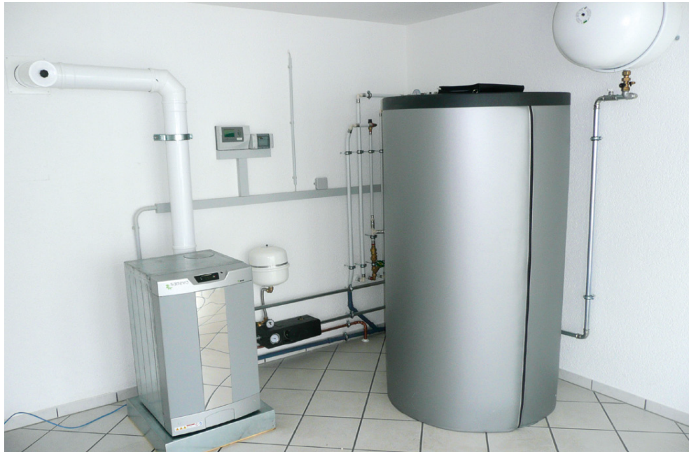
Figure 2.5: 1 kW WispherGen cogeneration system (adapted from Elmer et al. , 2015).
