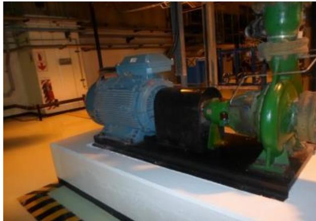
**Figure 2-2. An in-service pump coupled to its motor (normal image)**
