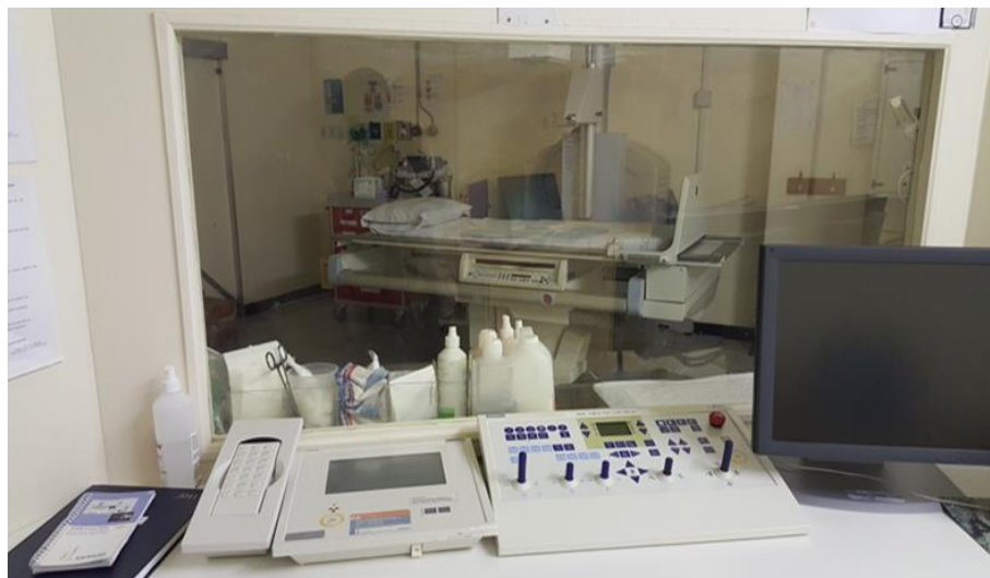
Figure 3.2: Siemens Iconos R200 Controls and display monitor at the research site
