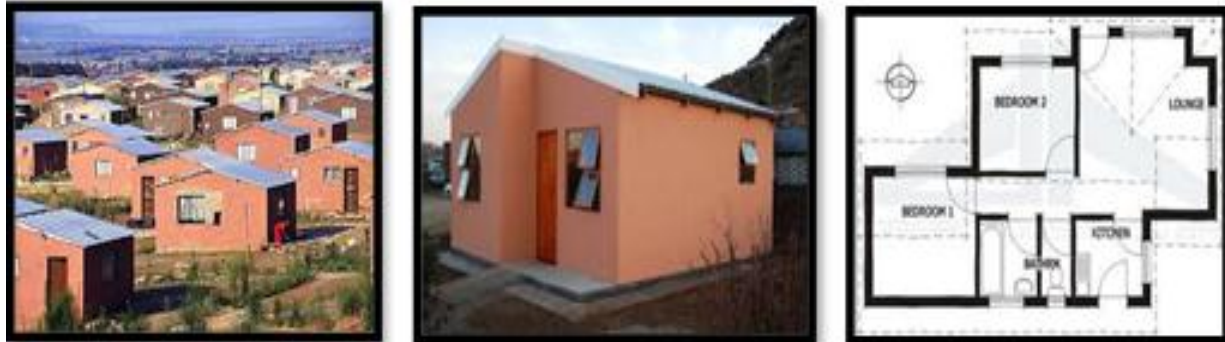
Figure 2.1 Typical two bedroom RDP house (Moladi, 2017)
