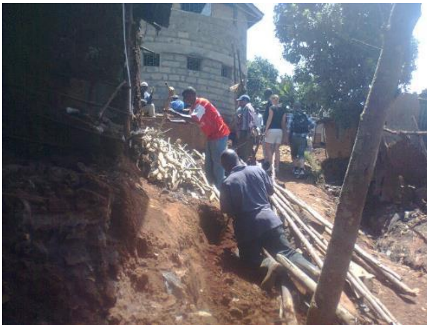
Figure 4.54: Construction of Biogas Centre in Kibera
