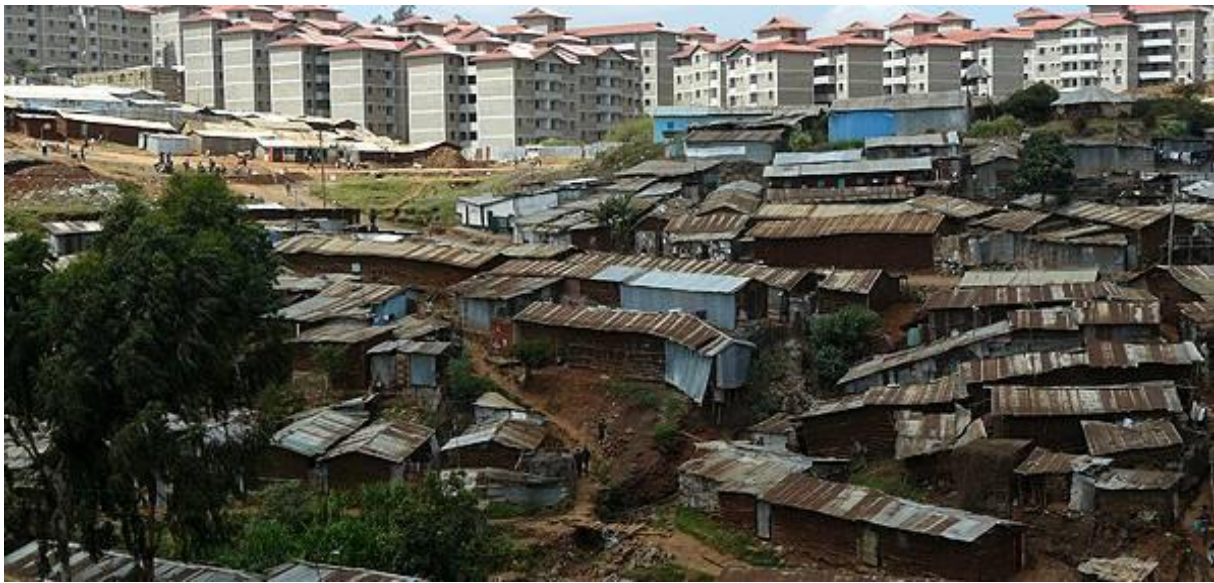
Figure 7.7: New housing project that is set to replace the adjacent informal settlement
