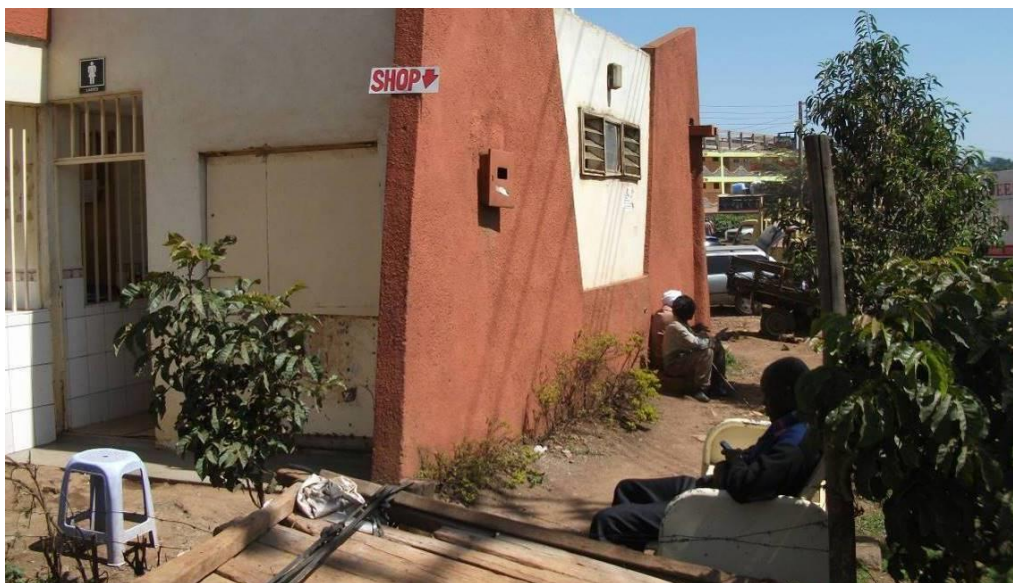
Figure 4.21: Side view of Iko Toilet at Limuru bus-stop showing community members at facility
