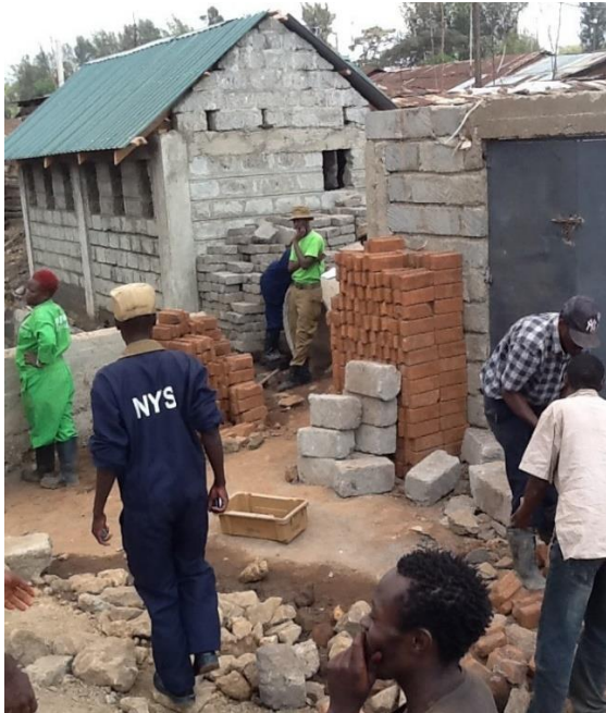
Figure 7.5: Construction of ablation blocks by NYS and volunteers in Kibera (Anon, 2014).
