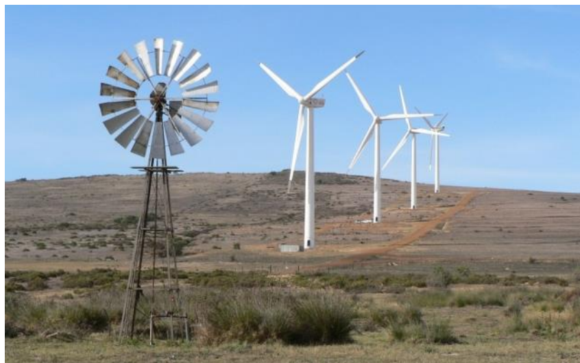
Figure 2.24: Darling Wind Farm (Darling windfarm, 2010)
