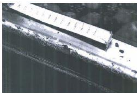
Figure 2.4: Spalling in rails [Rhen and Larsson, LTU]
