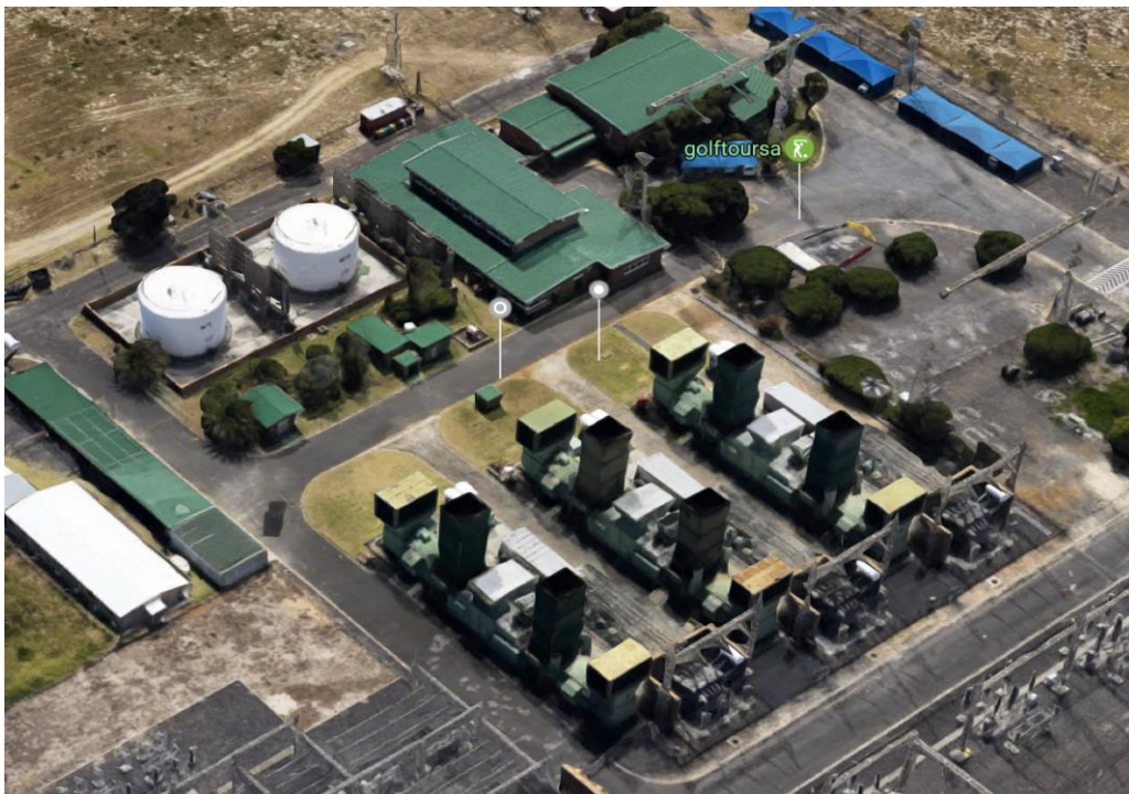
Figure 3.8: View of Acacia power plant (Source: Google Maps)
