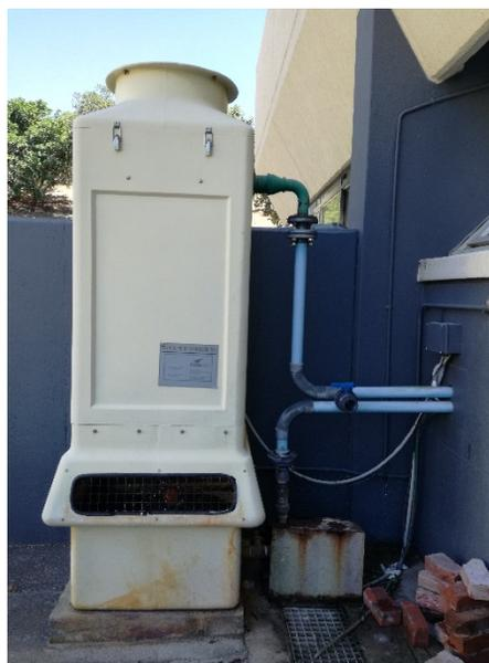
Figure 3.11: a) piping system that connects the chiller to various systems as well as the continuous re-circulating batch photoreactor b) chiller
