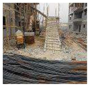
Figure 4.3: Abnormal way of piling materials on site
