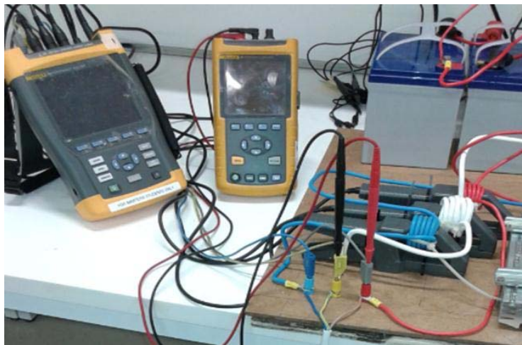
Figure 7-12: The Fluke 43B and Fluke 435B connections on the output side of the motor drive.
