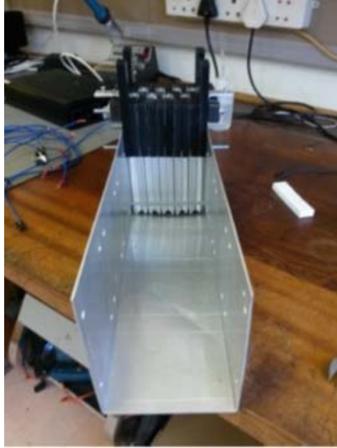
Figure 5-2: Assembly of aluminium enclosure for the battery pack
