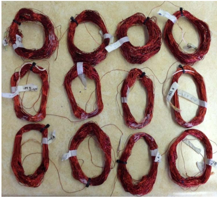
Figure 4-6: Original windings laid out for mapping
