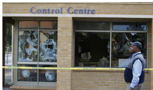
Figure 4.7: Damage done by protestors on campus 8: Damage done by protestors to classrooms (Bothma, 2016)
