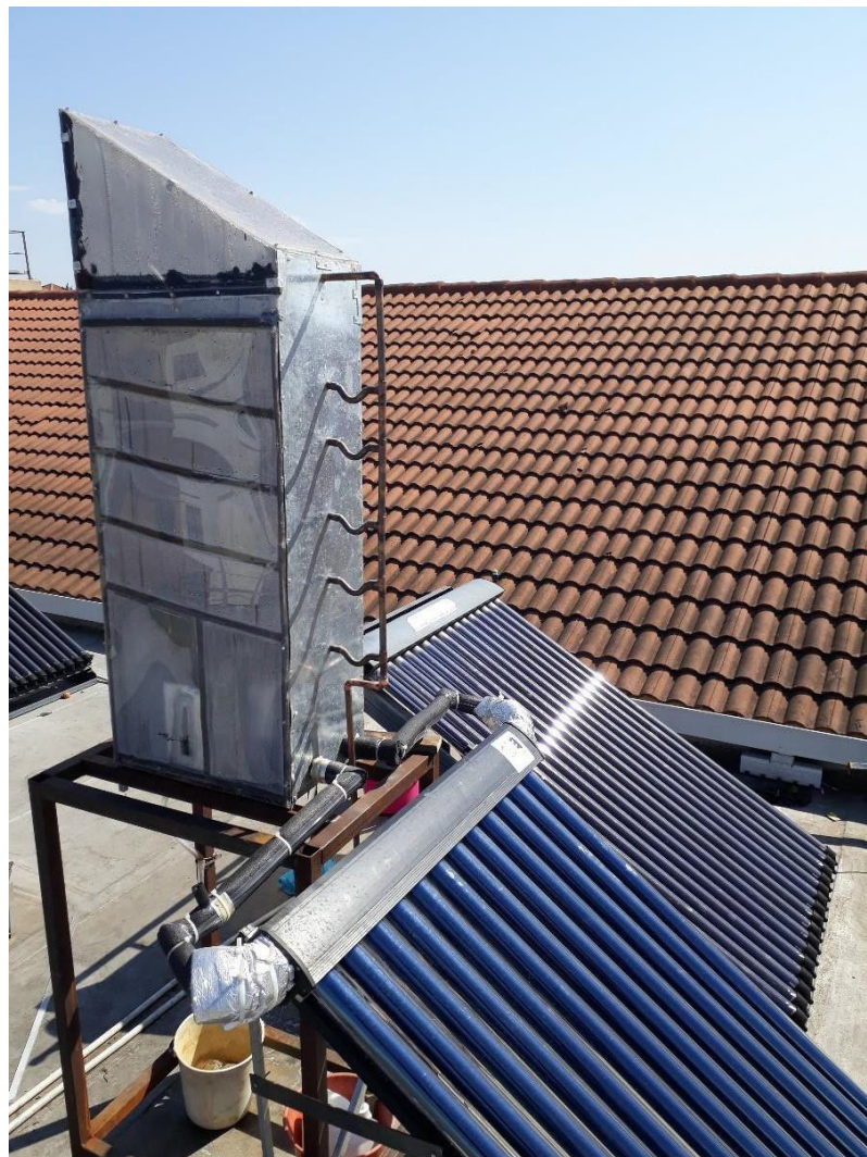
Figure 3.32: Multistage solar still desalination system
