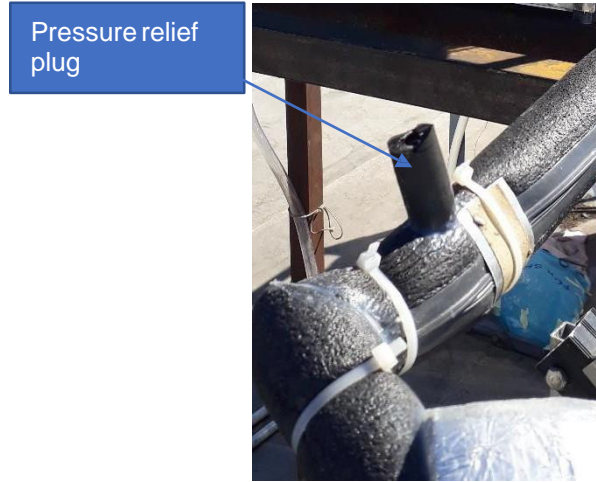
Figure 3.22: Pressure relief plug
