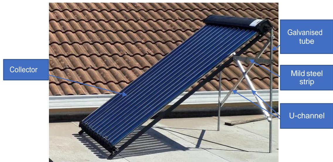
Figure 3.18: Evacuated tube solar collector at 33° from the horizontal
