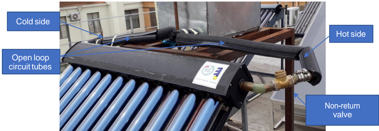
Figure 3.19: Open loop circuit and non-return valve
