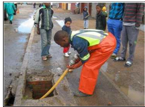
Blocked Drains Clearing
