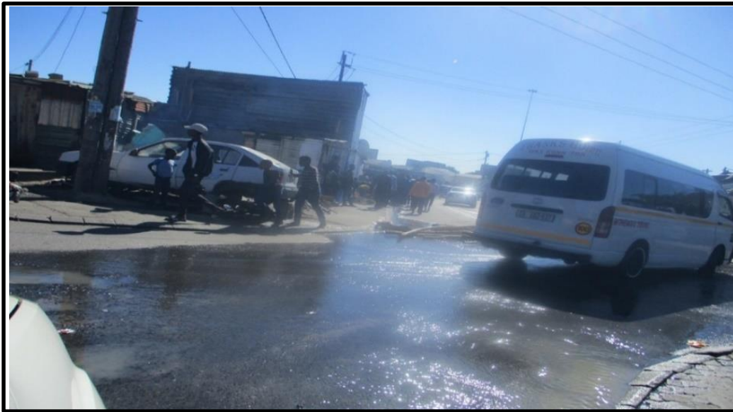
Figure 4.15: Blocked drains causing overspill of waste water in the public street
