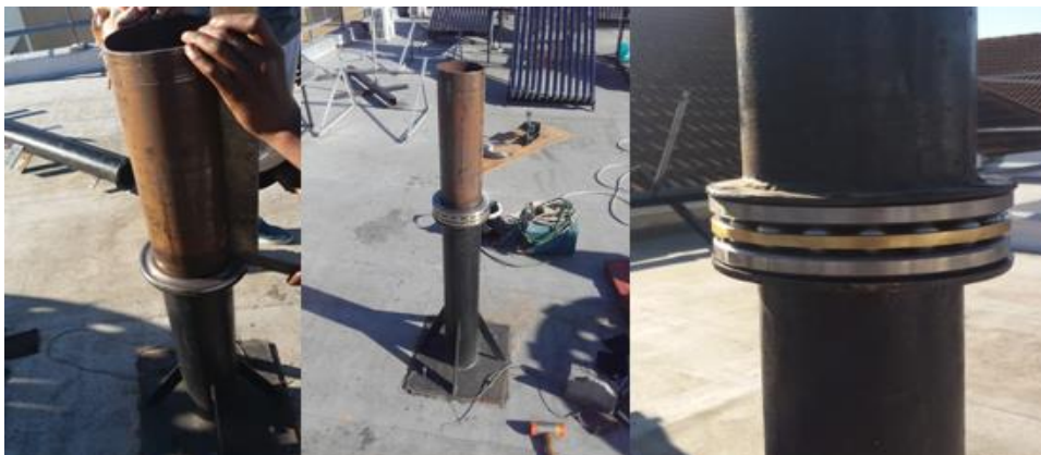
Figure 3.23: Bearing installation
