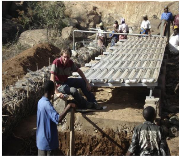
Figure 2.4: Solar water continuous disinfection (Mac Mahon & Gill, 2018)
