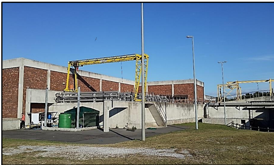
Photograph 3. 1: Full-scale MBR plant with six trains linked in parallel feeding the RO pilot-plant attached (left), biological reactor and the MBR submerged plant (right).
