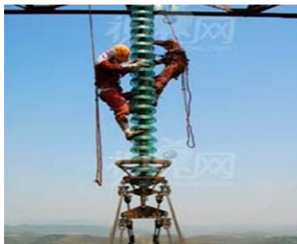
Figure 2-9: linemen cleaning insulators by hand wiping. (Wang, et al., 2016)
