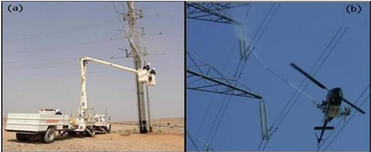
Figure 2-10: (a) Hot washing using a specialised truck. (Pressure washers pro, 2013) (b) Hot washing using a helicopter. (Red Eléctrica de España, 2008)
