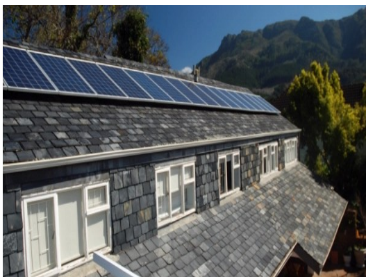
(a) Rooftop PV without structure
