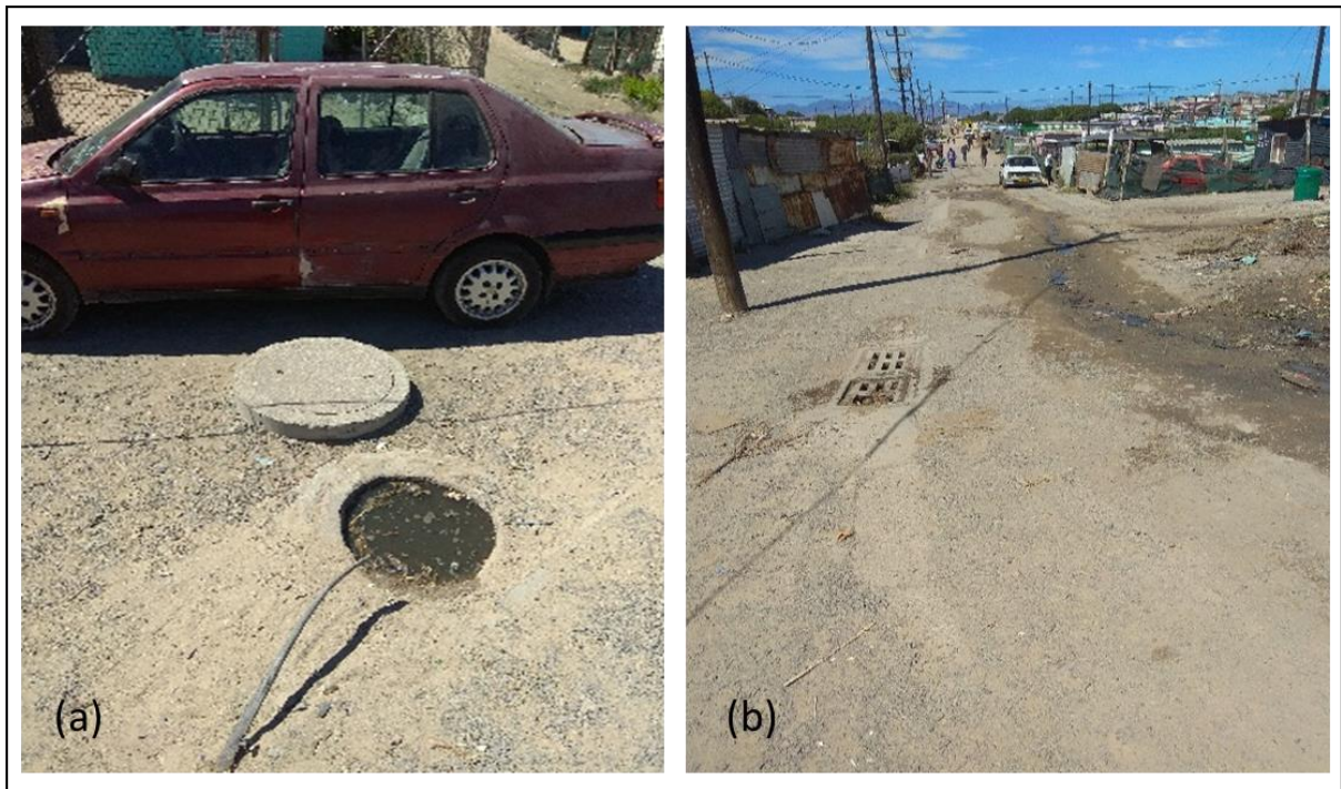
Figure 4:50 : Manhole and stormwater channel and kerb in-let.
