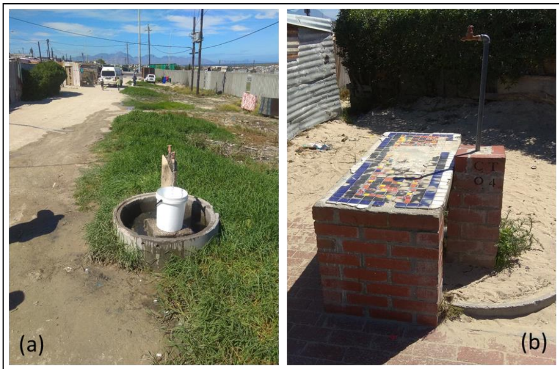
Figure 4:10: Communal standpipes.
