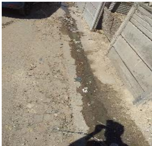
Appendix 13:(a&b): Photo a & b shows stormwater channels in which photo a has greywater runoff.
