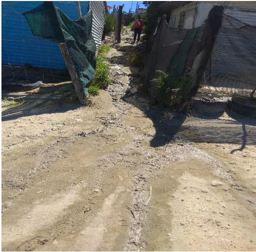
Appendix 11: (a&b) : Photo a shows greywater coming down the slope from a house in a much higher gradient and Photo b shows pondering of that greywater coming from up stream.
