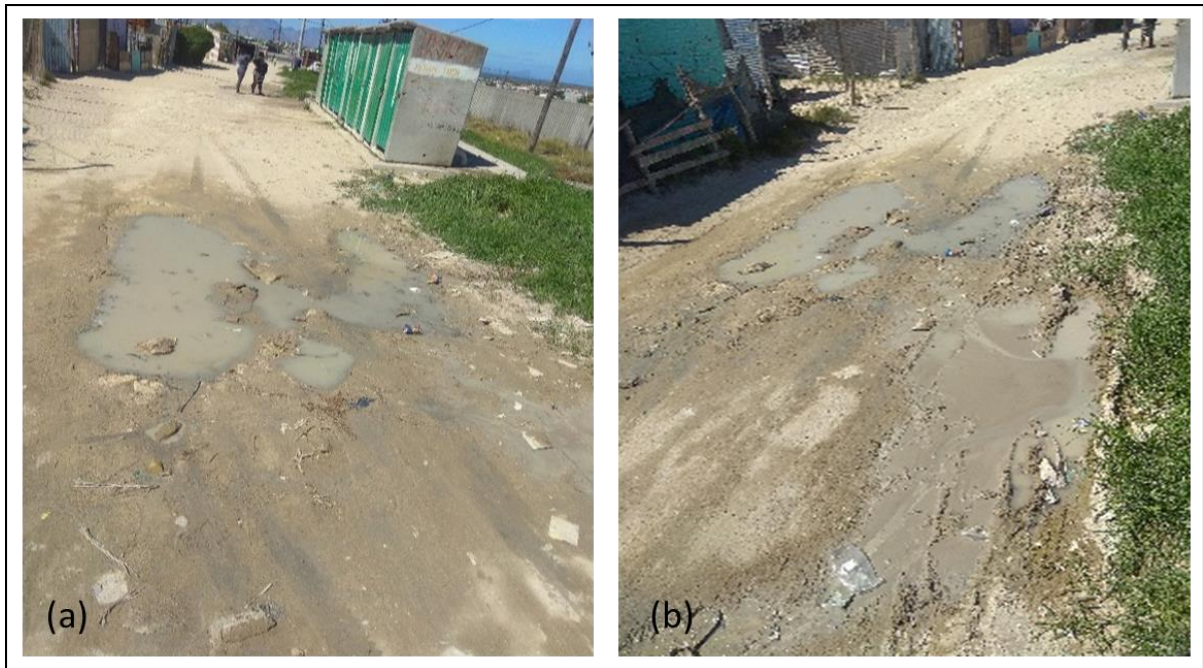
Figure 4:47: Ponding of greywater.
