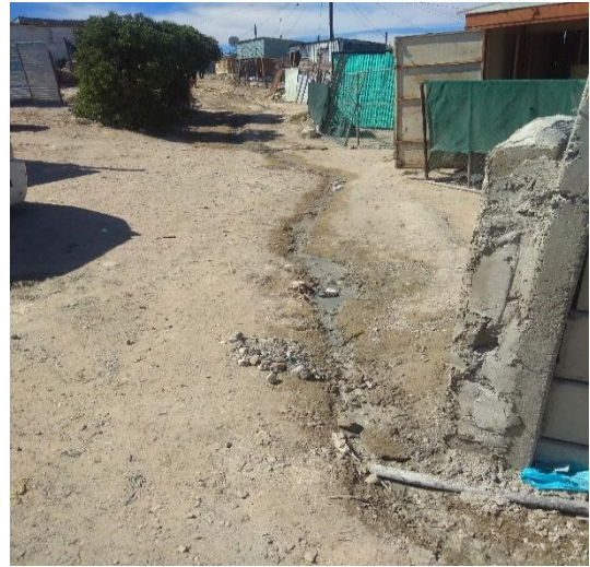
Appendix 11: (a&b) : Photo a shows greywater coming down the slope from a house in a much higher gradient and Photo b shows pondering of that greywater coming from up stream.
