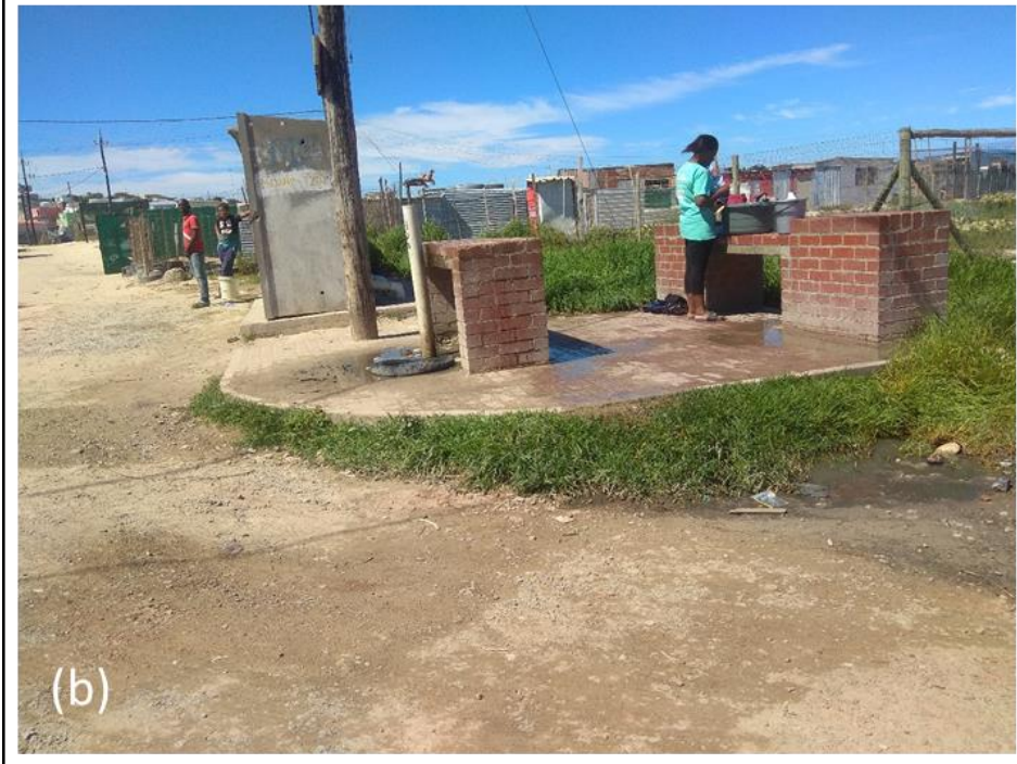
Figure 4:52 : Emthonjeni facilities in section B and C.
