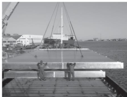
Figure 1.3: FSW deck panels for cruise ship [Gordon, 2010]
