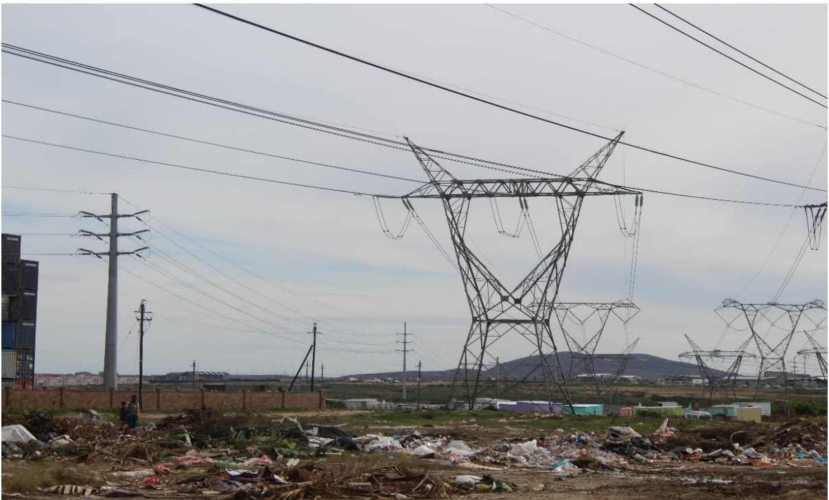
Figure 4.4: Illegal Dumping Site close to Dwellings
