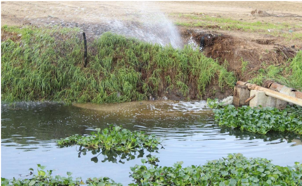
Figure 4.15: Raw sewage entering Diep river due to pipe burst
