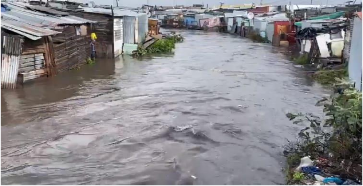
Figure 2.4: Flooding in Kosovo informal settlement, Philippi, Cape Town (SABC News, 2020)
