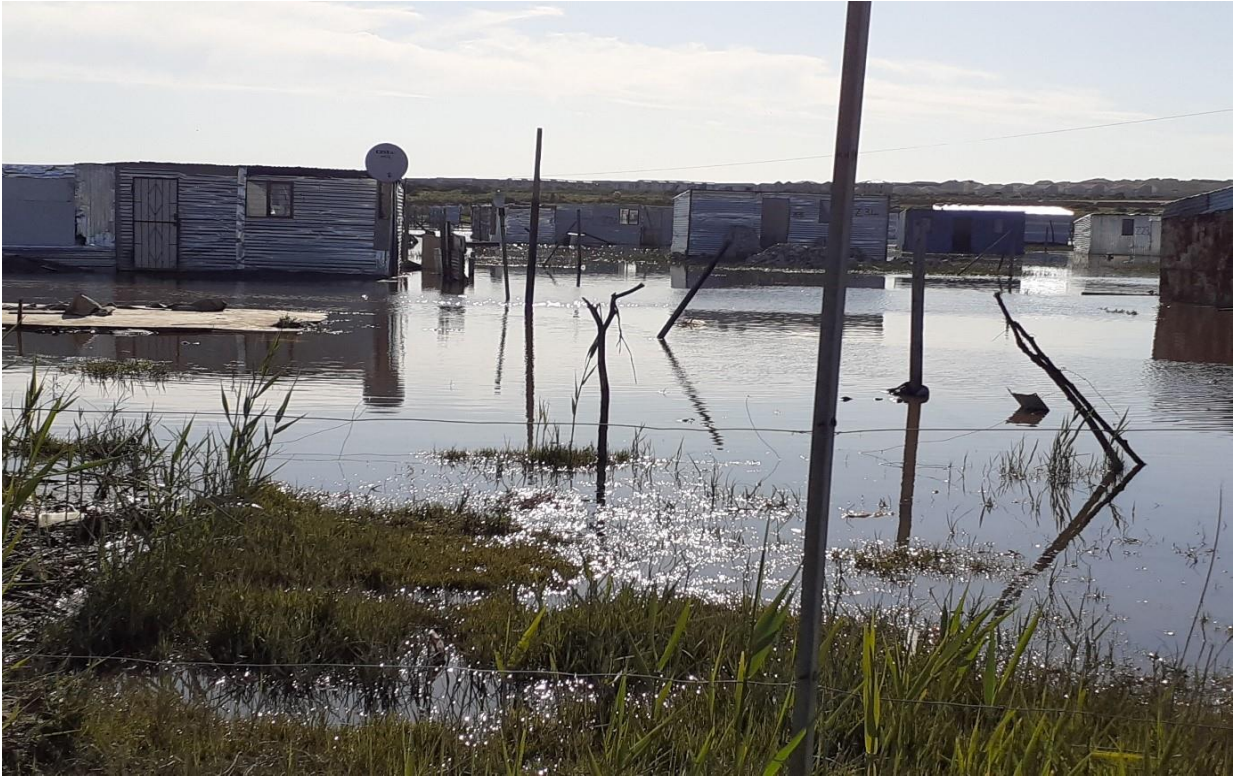
Figure 4.13: Flooding in Dunoon Informal settlement, Zwezwe
