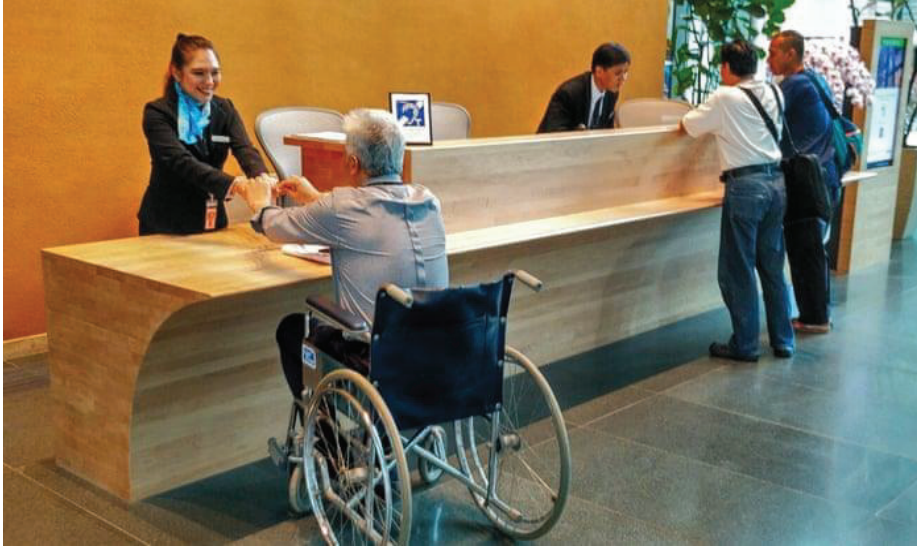
Figure E.12: Lowered reception desk for wheelchair travellers (Source: The Guardian, 2019)
