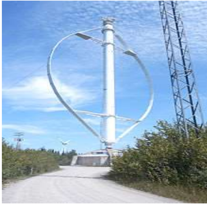
Figure 2. 19: Vertical wind turbine position (Hemami., 2012)
