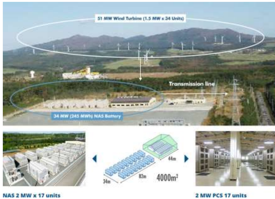
Figure 4-3: A sample of 51MW and 34MW capability built-in NAS with a capability of 245 MWh (Zareifard, 2017).
