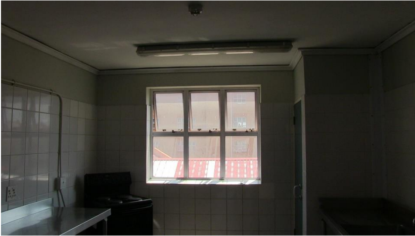
Figure 4.11: Kitchen area showing lamp fittings, sink and stove.
