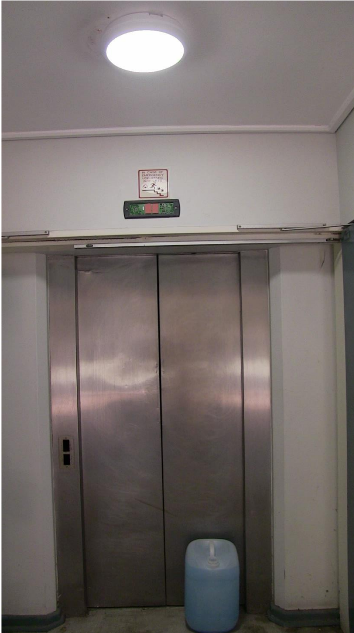
Figure 4.20: Elevator at Catsville
