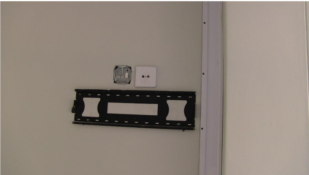
Figure 4.19: Socket outlet and TV mounting bracket
