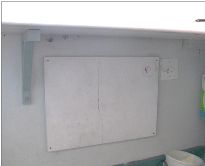
Figure 4.6: 400W panel heater (wall mounted)
