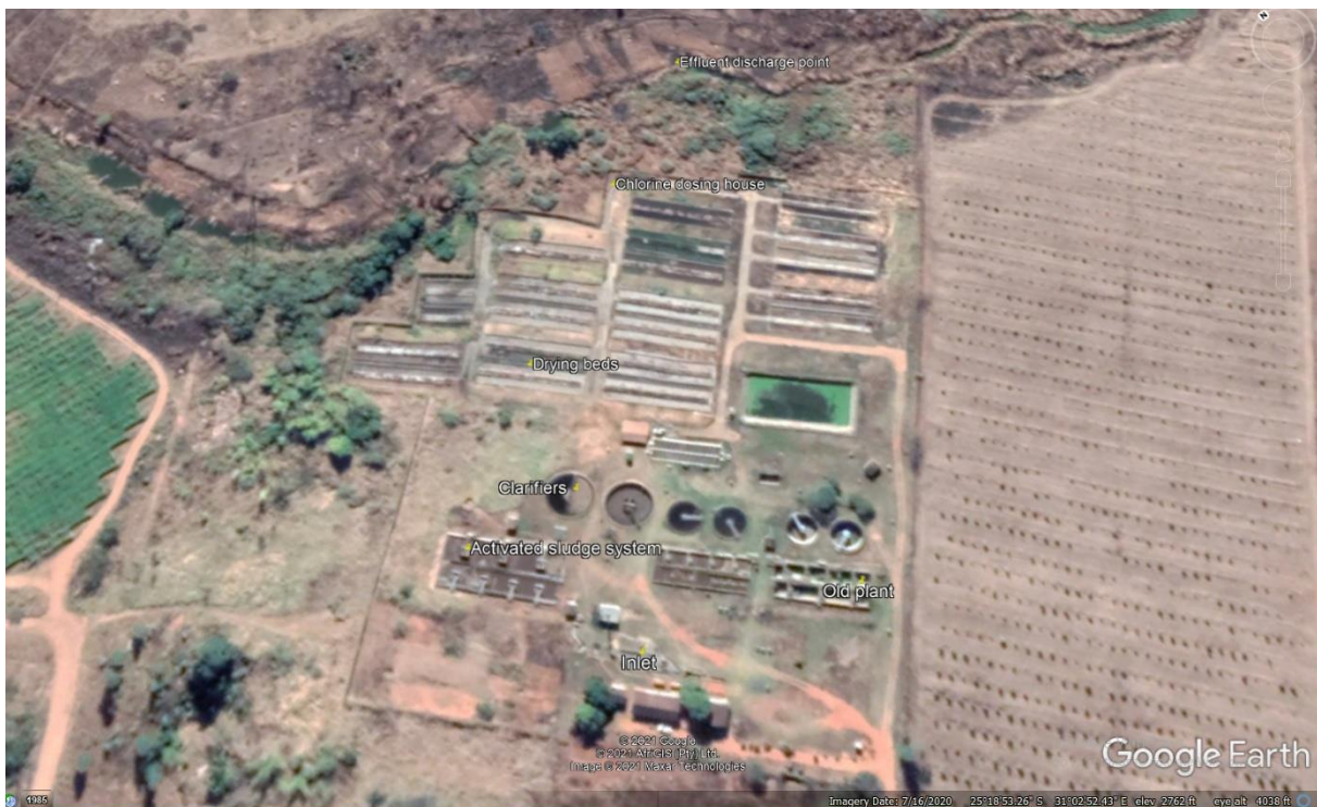
Figure 4.13: A google image showing the location and layout of White River WWTW (google earth, 2021)
