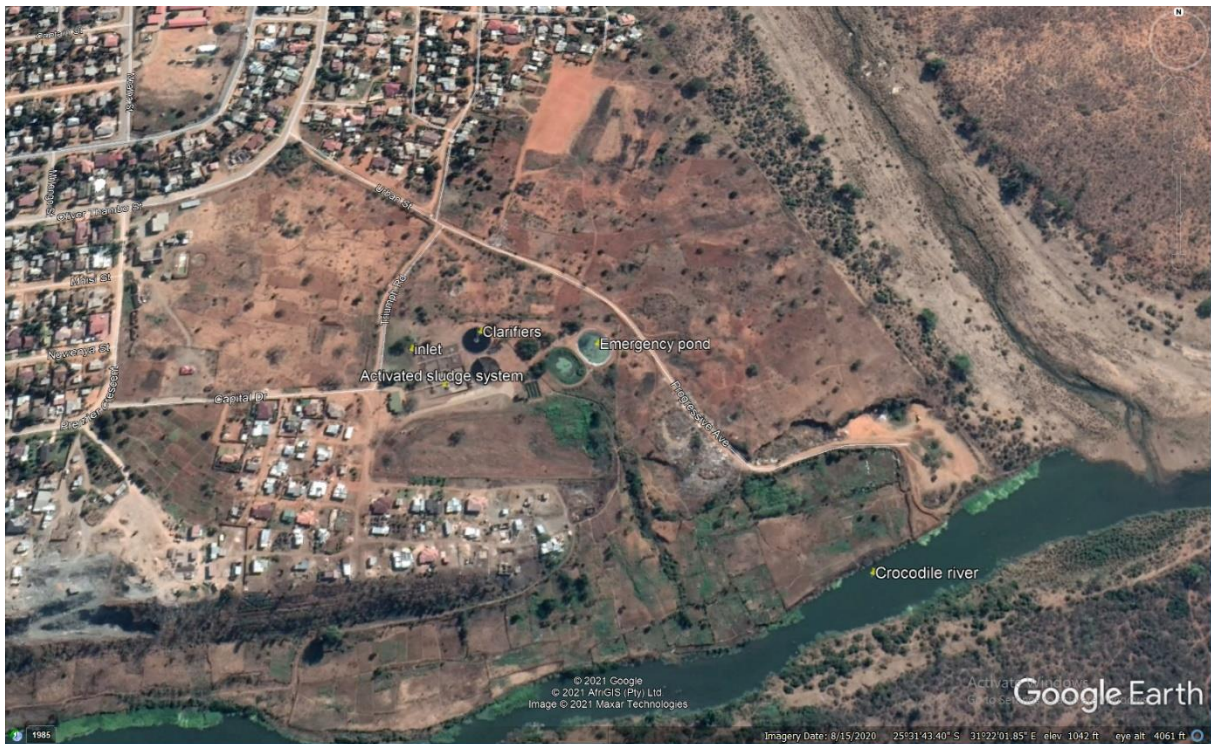
Figure 4.17: A google image showing the location and layout of Matsulu WWTW (google earth, 2021)
