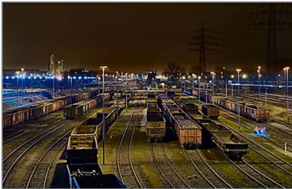
Figure 2-1 (a): Sentrarrand freight rail shunting yard at night
