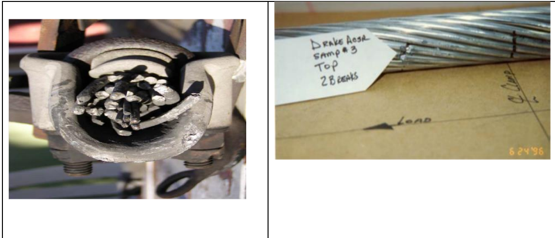
Figure 2. 2: ACSR Fatigue Failure & Broken Aluminium Strands (Alderton et al., 2015)
