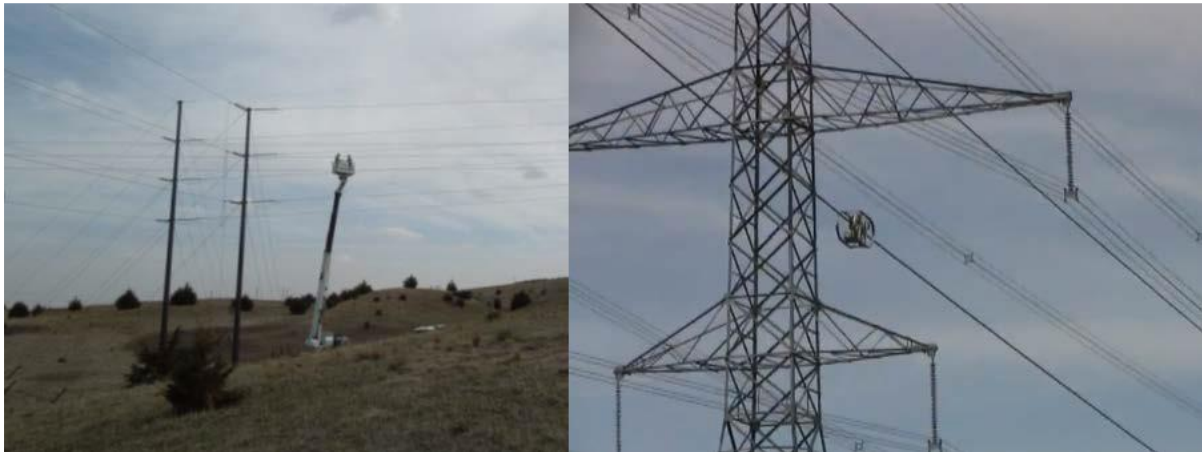
Figure 2. 4: Transmission line electromagnetic testing (Wayer, 2016)
