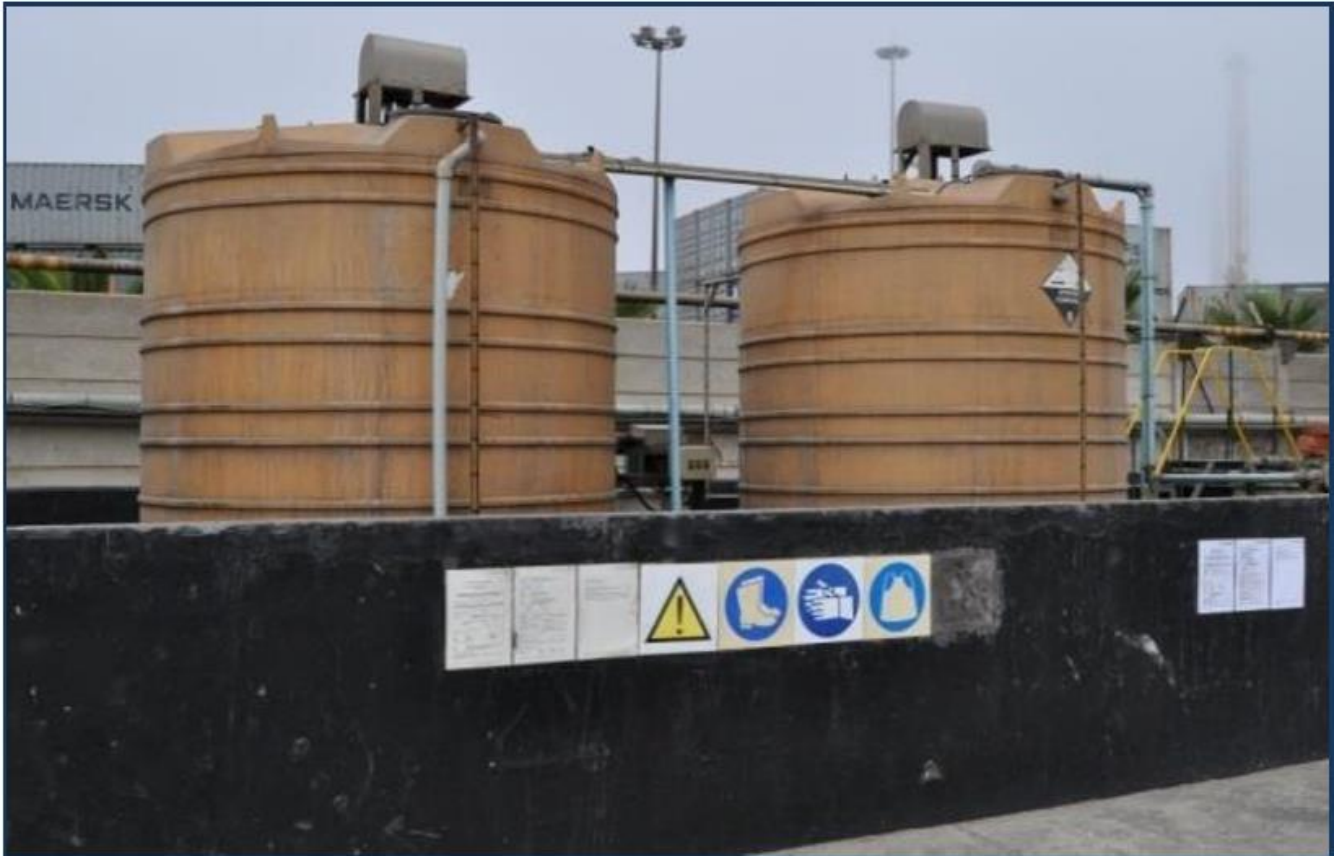
Figure 2-2: Coagulant and flocculent chemical dosing tanks at the fish factory (Source: Geo Pollution Technologies 2004)
