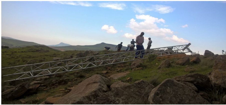
Figure 2 – Remote site pre-installation
