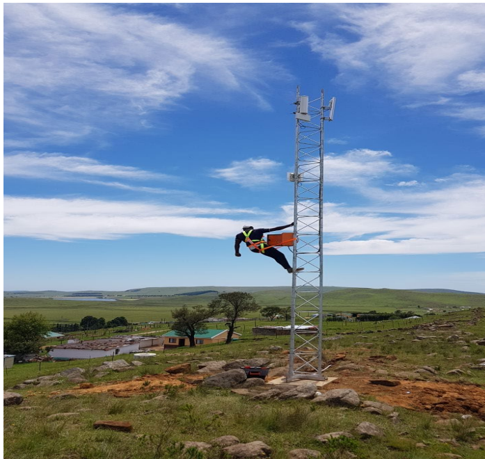
Figure 4 –Remote high site installation for broadband services
