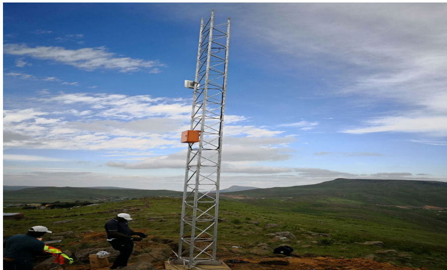
Figure 3 – Remote site post- installation
