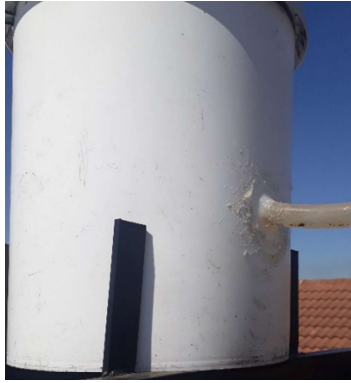
Figure 3.7: External saline water tank
