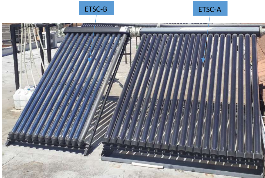
Figure 3.76: Evacuated tube solar collectors
