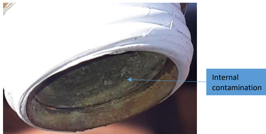
Figure 5.51: Non-return valve contamination
