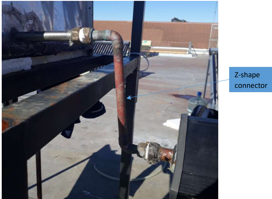
Figure 3.80: Z-shaped tube connection
