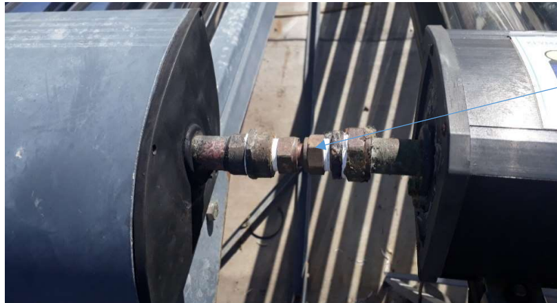
Figure 3.78: ETSCs connected in series
