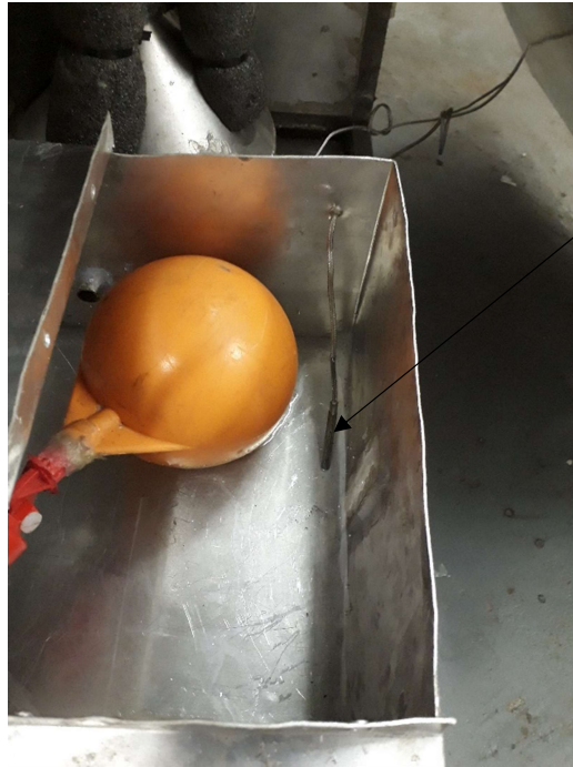
Figure 4.9: Liquid probe inside the secondary SW tank
