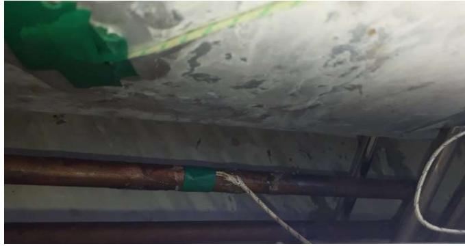
Figure 5.49: Stage 2 trays and zigzagged SW tube
