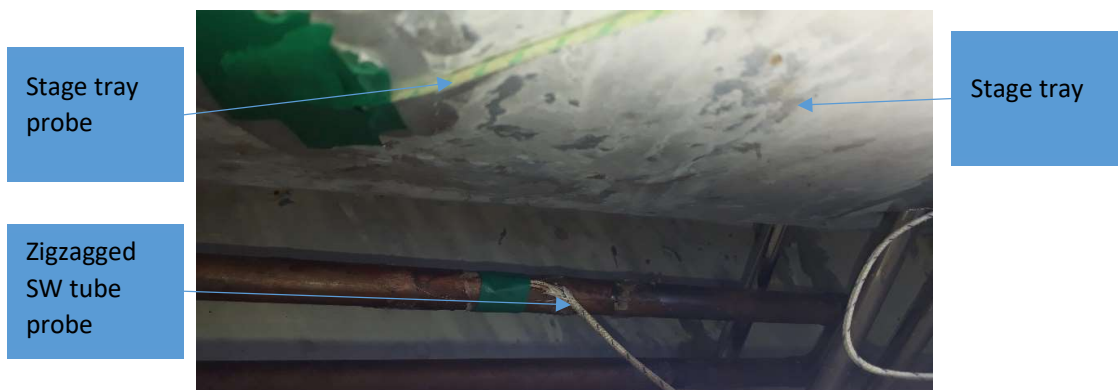
Figure 4.11: Surface probes attached to the zigzagged SW tube's outer surface
