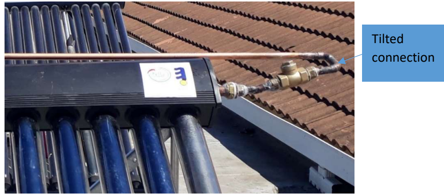
Figure 3.74: Tilted end connection
