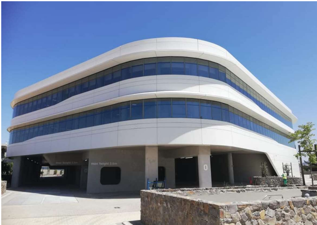
Figure 24: Capitec Bank head office site view 3 (Capitec, 2021)
