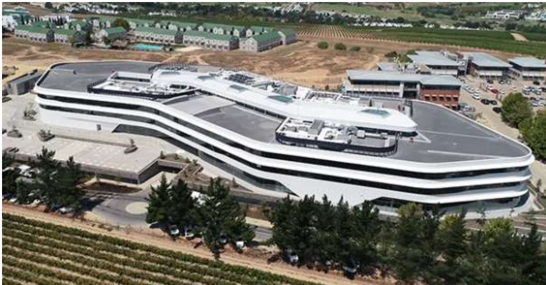
Figure 22: Capitec Bank head office panoramic site view 1 (Capitec, 2021)
