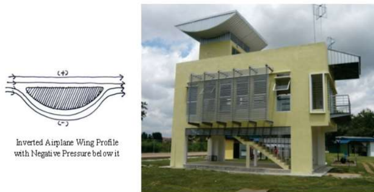
Figure 5: Wind-induced experimental house (Haw et al., 2012)
