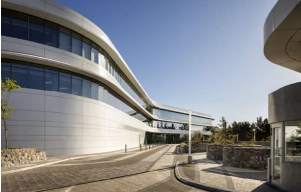
Figure 23: Capitec Bank head office site view 2 (Capitec, 2021)
