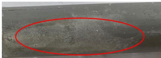
Crazing, material erosion and discoloration
