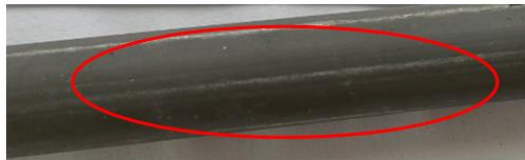
Dry band activities on the surface
