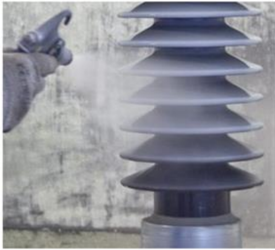
Figure 2-5: Spray painting of high-voltage insulator with RTV-SR coating
