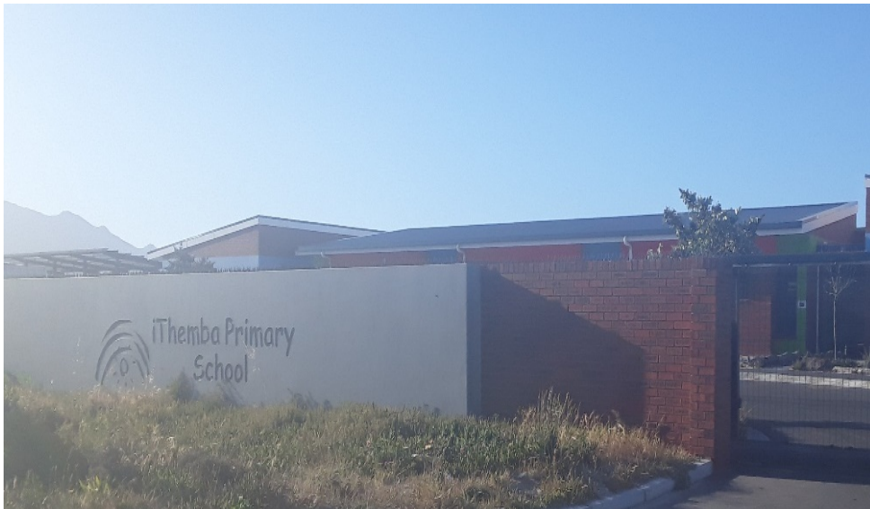
Figure 4.32: Second primary school (iThemba primary school) in Capricorn Park, as demand rises
