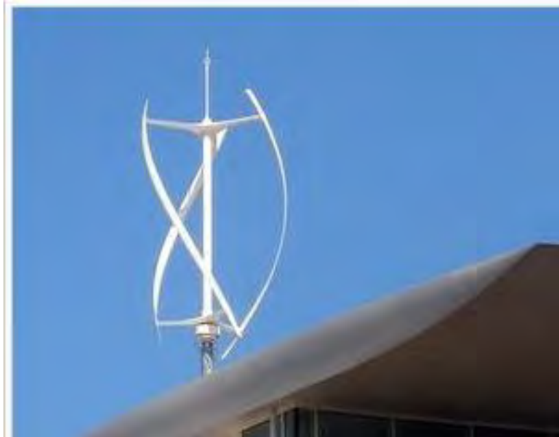
Figure 2.4: Typical Vertical Axis Wind Turbine (WED, 2015)
