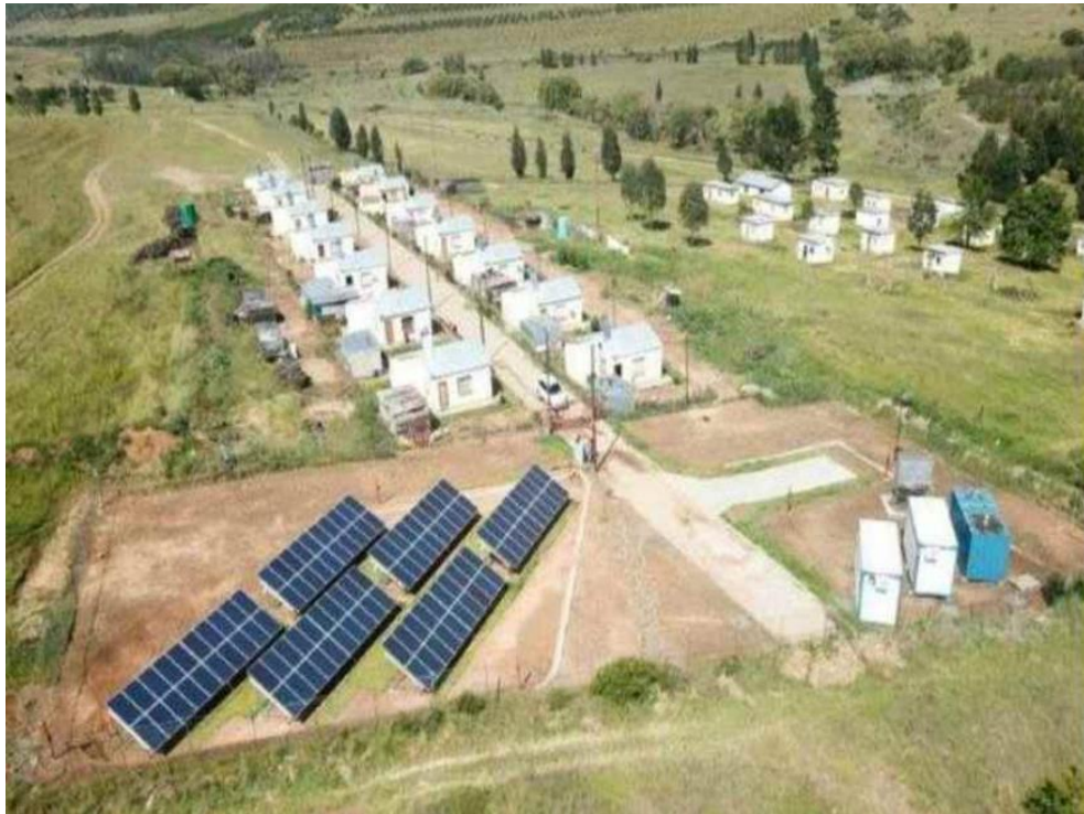
Figure 6. 4: Wilhelmina solar microgrid, Ficksburg – SA (Zyl, 2018)
