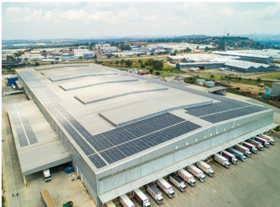
Figure 6. 6: Grid-tied Solar PV microgrid, Johannesburg – SA (Published with permission from SOLA group)
