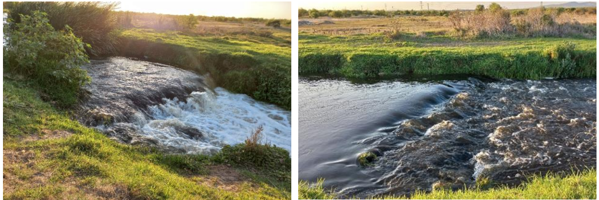
Figure D.1: ZWWTW canal from the road to the river
