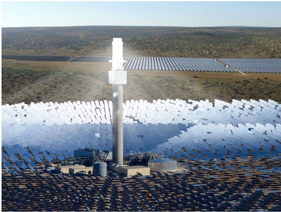
Figure 2.13: The Redstone concentrated solar power plant in the Northern Cape, South Africa (From NS ENERGY, 2018)
