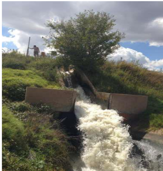
Figure 2.31 Rooiwal Wastewater Treatment Works outlet in South Africa (From Loots et al., 2015)
