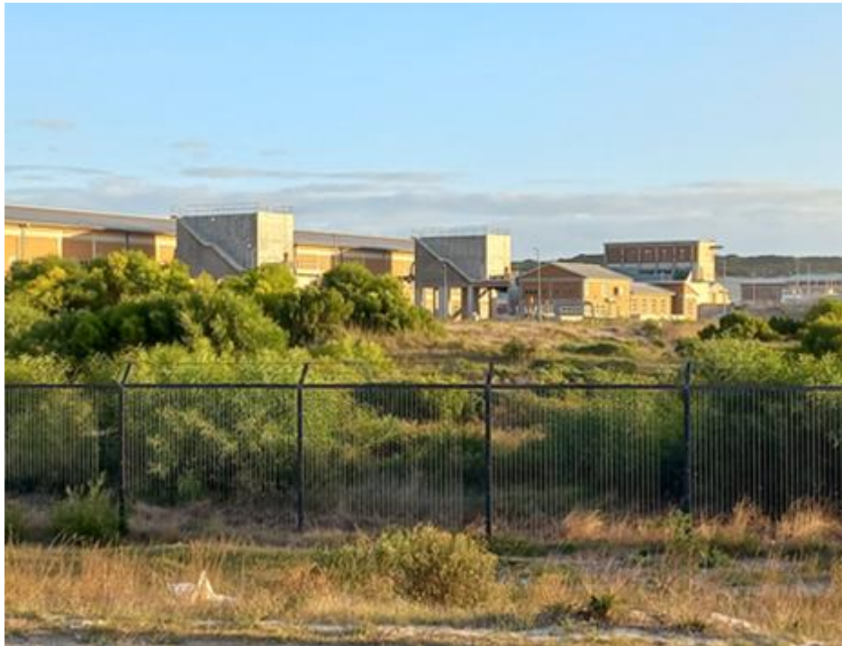
Figure D.2: View of the ZWWTW from the road
