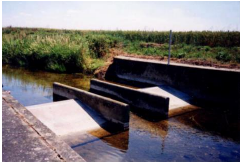
Figure 3.14: Example of a river weir (Rickard et al., 2003)
