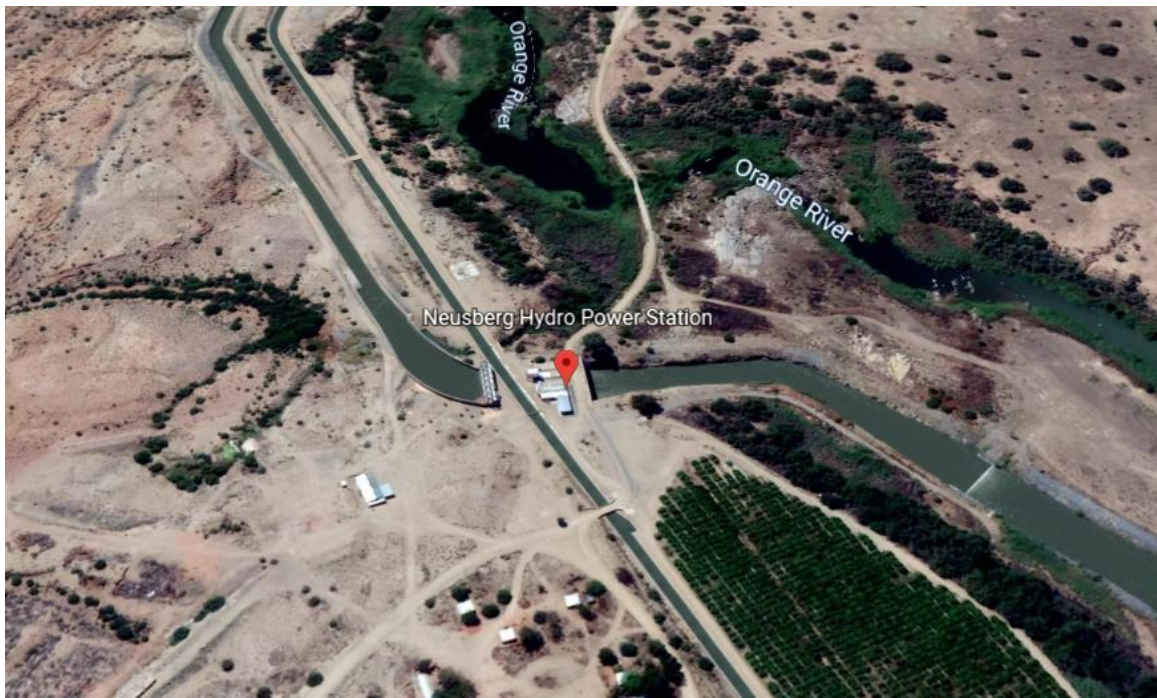
Figure 2.18: Location of the Neusberg small hydropower station on the Orange river in the Northern Cape in South Africa (Adapted Google Maps, 2021b)
