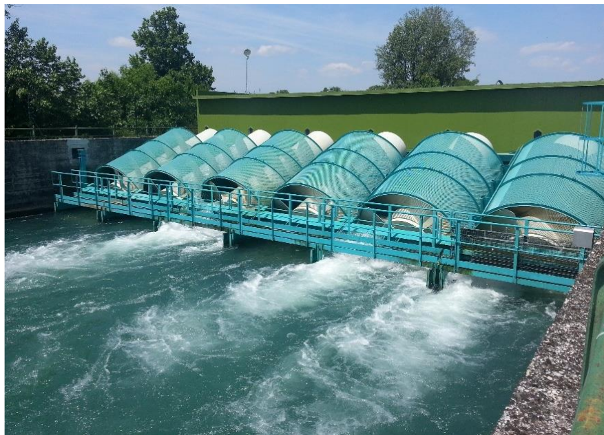
Figure 3.5: Archimedes screw turbine (From HydroSmart, 2021)
