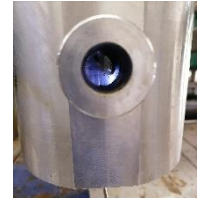
Sight glass (located on samp)
