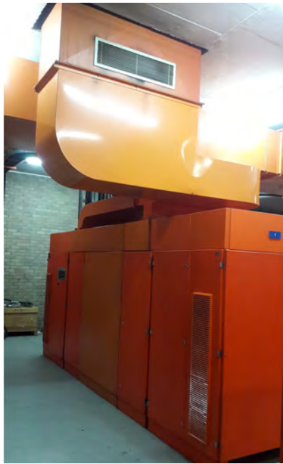
Figure 2.3-2: Air circulation system
