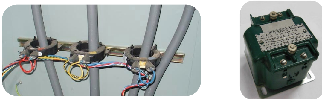
Figure A.3: Instrument transformers, left-to-right: current transformer, and voltage transformer (Ali@gwc.org.uk, 2004; Wordtwist, 2013). CC BY-SA 2.5 , CC BY-SA 3.0
