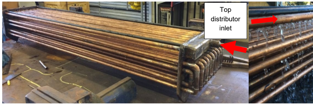
FIGURE 3.5: EVAPORATOR HEAT EXCHANGER
