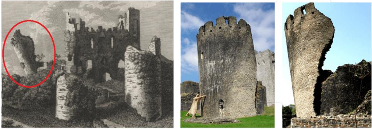
Figure 2.27: Artist drawing of the leaning tower of Caerphilly Castle (left) and modern photos of the tower (middle and right) (D'Altri et al., 2018)
