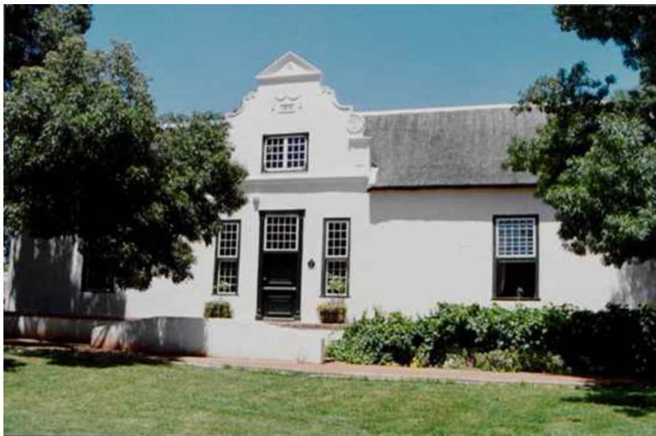
Figure 2.50: Front view of the Non-Pareille manor house
