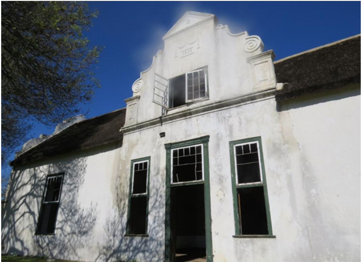
Figure 3.7: Non-Pareille manor house front gable (Van der Walt, 2016)
