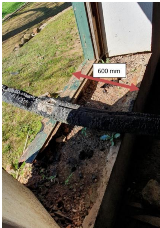
Figure 3.13: Wall width measured at the window opening
