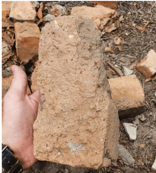
Figure 4.3: Masonry brick from old wall
