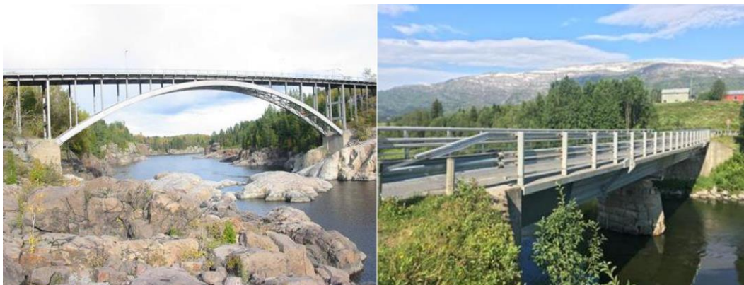
Figure 1.2: Arvida and Forsmo bridges [36]
