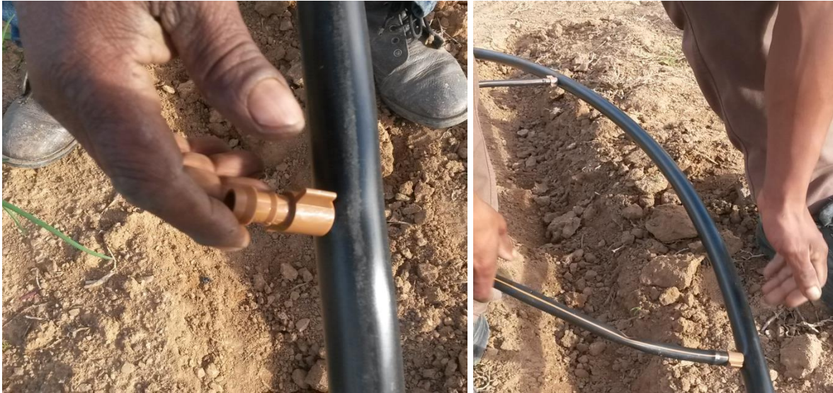
Figure 3. 7: Installing the dripper lines.
