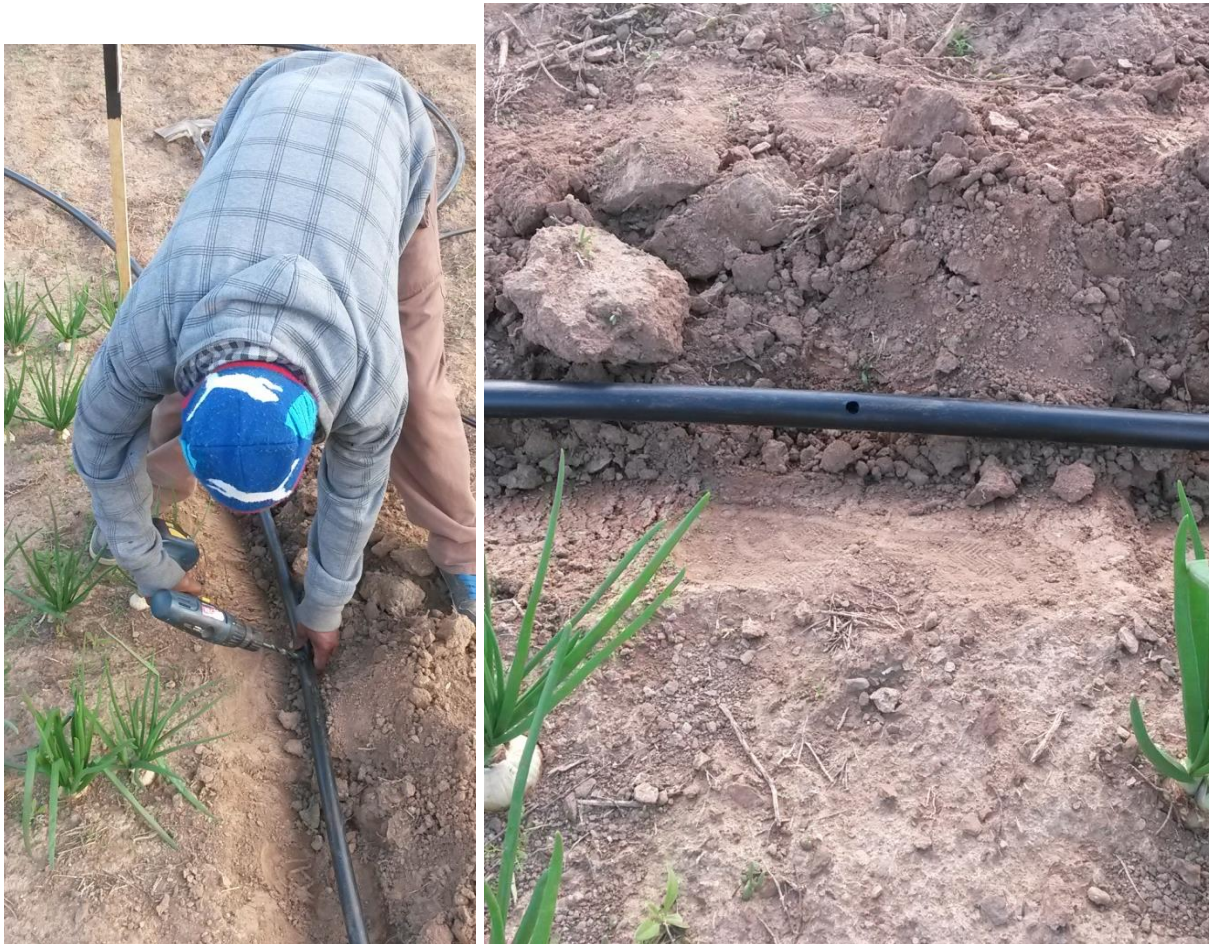
Figure 3. 6: Drilling holes in sub-line to connect the dripper pipes.
