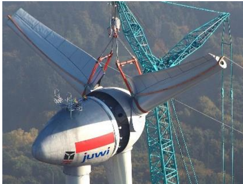
Figure 1.6: Steel blade stubs attached to hub of Enercon E-126
