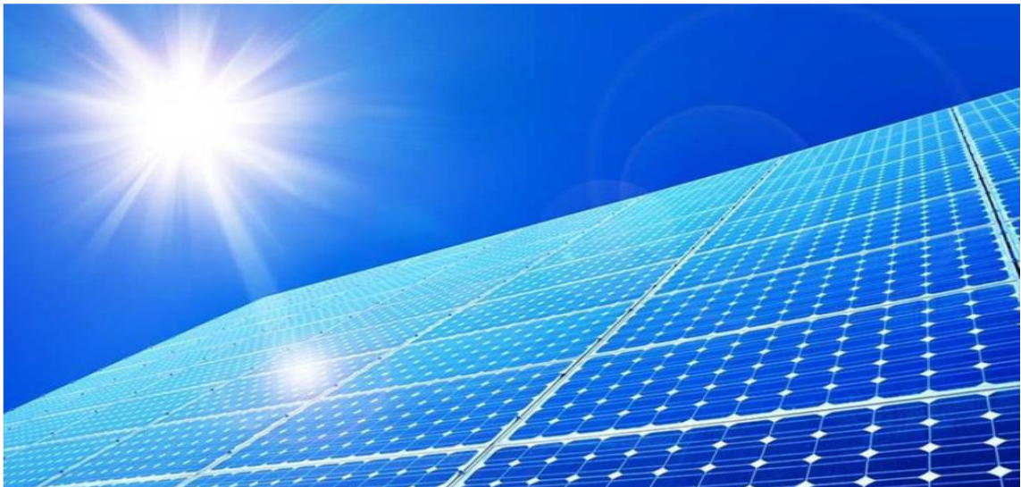
Fig. 2. 4: Photovoltaic Plant (Anon, 2020)
