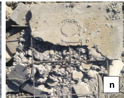
Steel measurement from the demolished panel (U)
