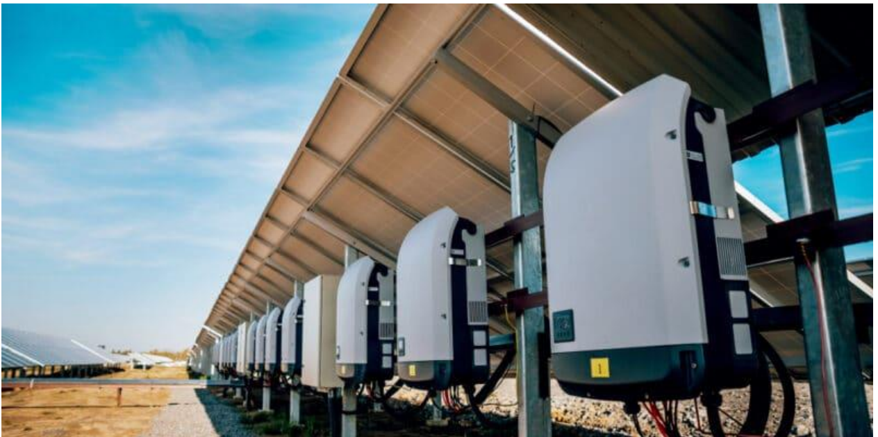
Figure 3.3.2.1: Inverters that are used in solar PV power plants. [27]
