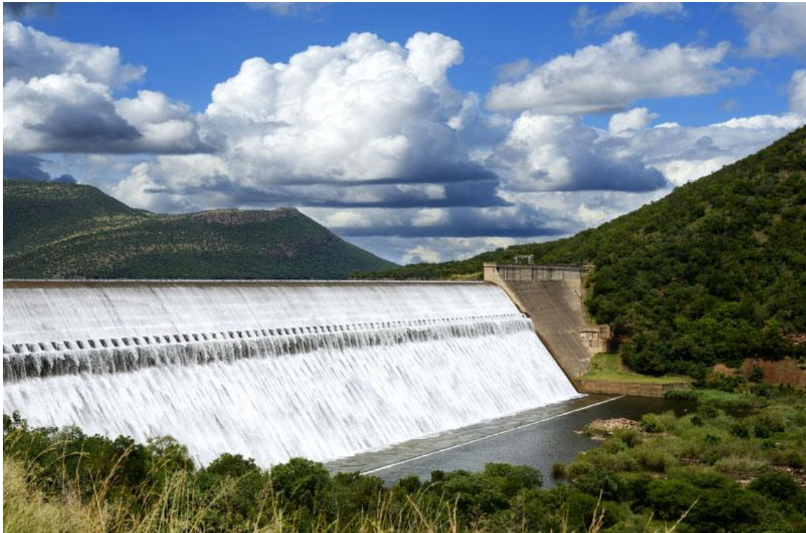
Figure 4.2.2.1: The Loskop Dam [32]
