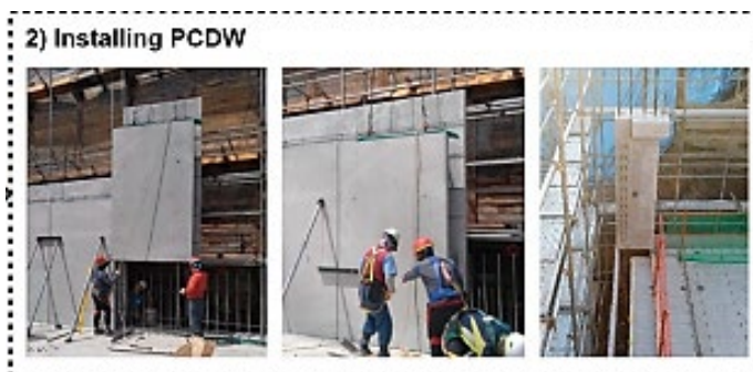
Figure 2.1 An illustration of a typical construction of a building panel (Kim et al., 2020)
